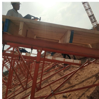
Operating Surface Installation 操作面安装
