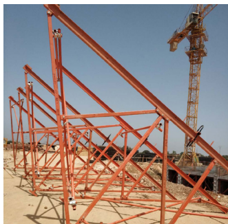
Steel Frame Installation 钢框架安装
